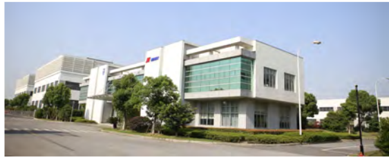
NEWAY Foundry (Suzhou) Founded in 2008 Main products: Sand Casting Expanded in 2015 Building area: 112,500 sqm Work shop: 98,000 sqm
